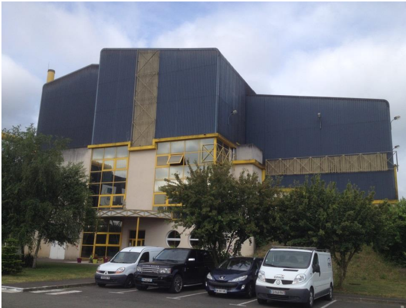
Figure 6 Energy from waste plant in Pontenx-les-Forges.
