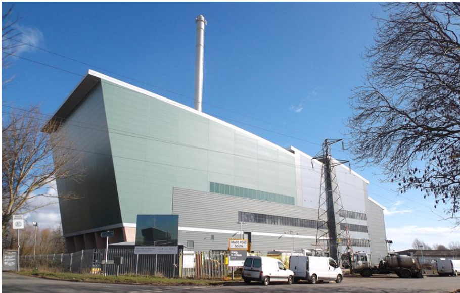
Figure 5 Exeter Energy Recovery Facility (Devon County Council).
